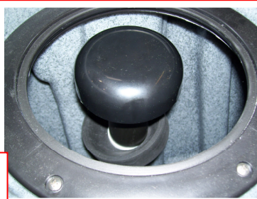
Float Shutoff Assembly
